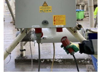
3 Disconnect the power cable.
